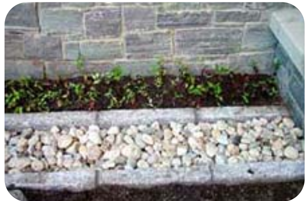
French Drain ©JES Construction, Inc.
