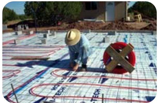
Laying Radiant Heating Pipes ©Melinda Honn
