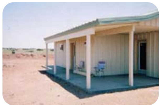
Covered Exterior Walkway ©Joel Kapp
